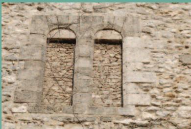
DEUX PHOTOS DE DÉTAIL COMPARÉES DE FENÊTRES GÉMINÉES DE LA FAÇADE OUEST, UNE AUTHENTIQUE, AVEC COUVREMENT MONOLITHE, UNE AUTRE DE 1882 AVEC SEULEMENT UN JAMBAGE (À DROITE) ANCIEN ET UN COUVREMENT EN PLATE-BANDE APPAREILLÉE
